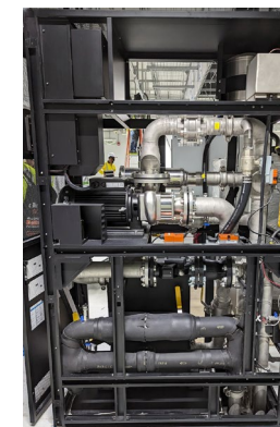
CDU internal components
